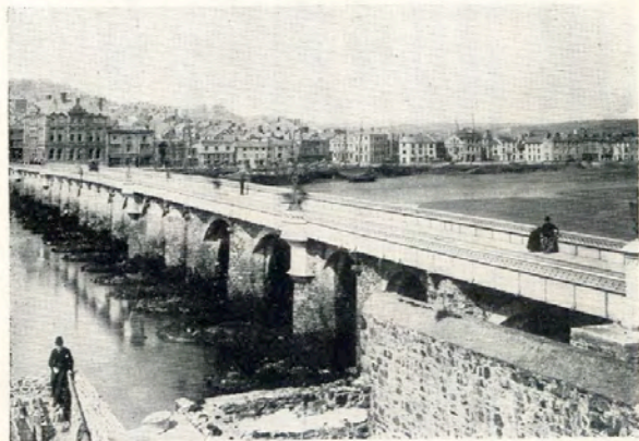
As it appeared prior to the last widening in 1925. (See page 28 for view of the famous Long Bridge as it is to-day).
