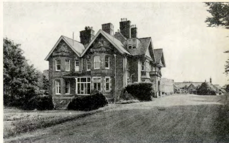
LAKENHAM, SENIOR RESIDENTIAL HOUSE
