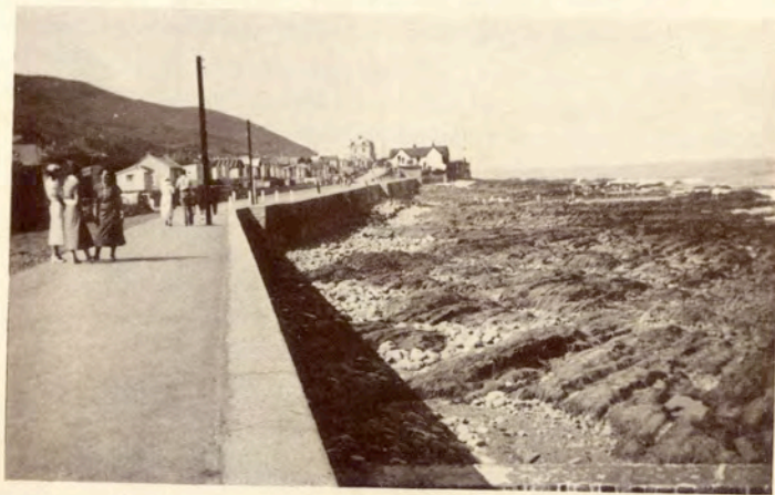
PROMENADE AND RAISED BEACH, WESTWARD HO!
