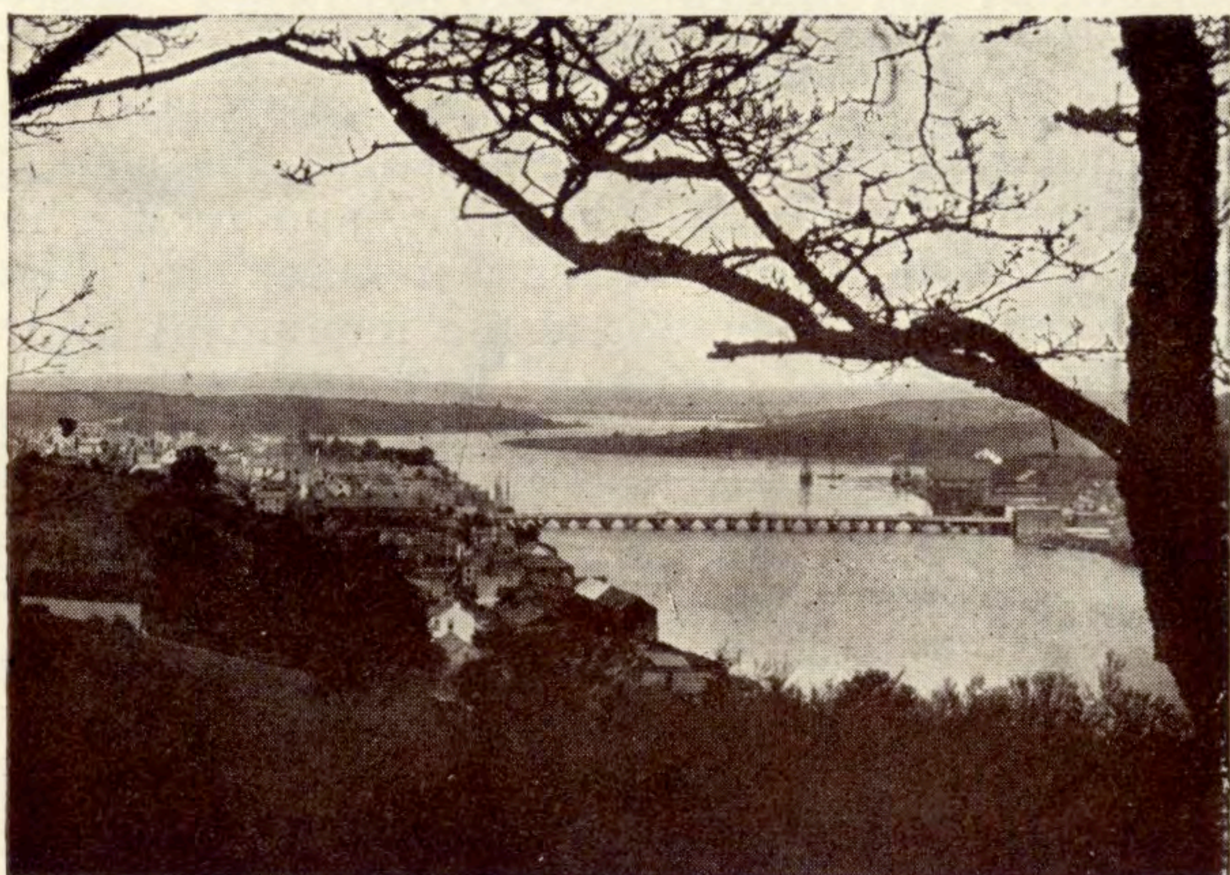
A VIEW OF THE LONG BRIDGE AT BIDEFORD
