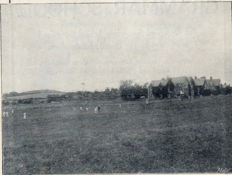
THE SCHOOL BUILDINGS AND CRICKET FIELD.
