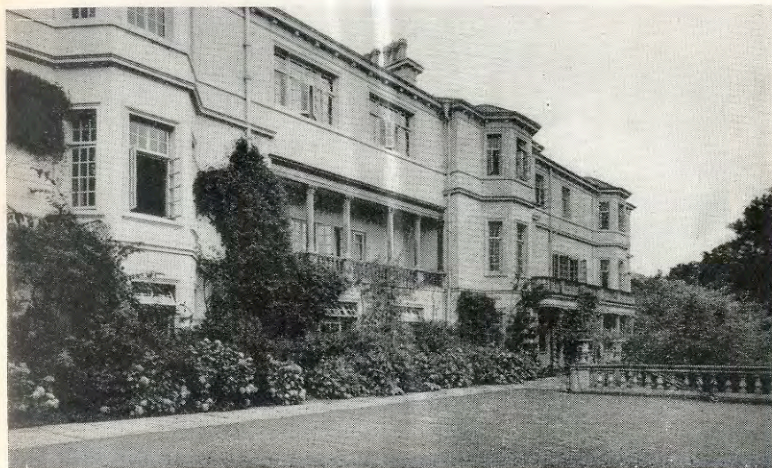
LAKENHAM, SENIOR RESIDENTIAL HOUSE
