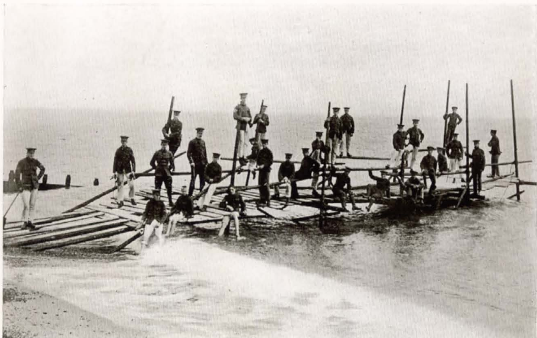
EASTWARD HO! TRESTLE BRIDGE BUILT BY THE COLL. CADET CORPS AT LANDGUARD FORT, FELIXSTOWE, AUGUST, 1907.
